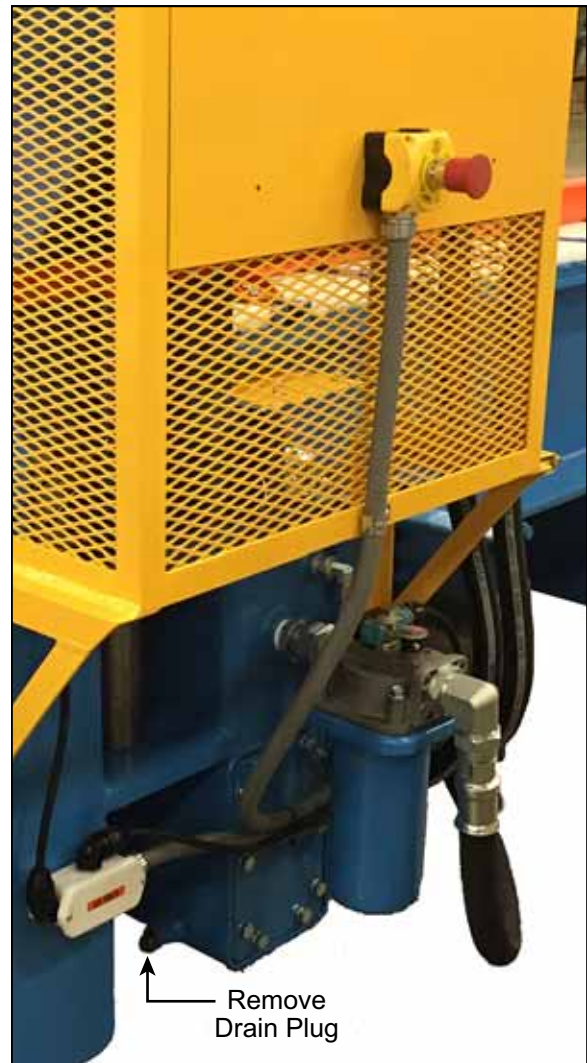
Figure 7-6: Draining the Reservoir
